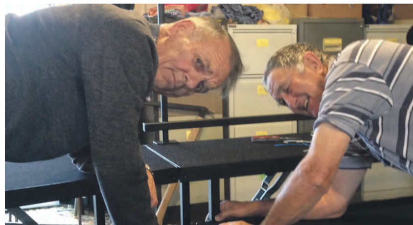
Stratford Singers' Bernard Hughes and John Sextus constructing new choir risers
